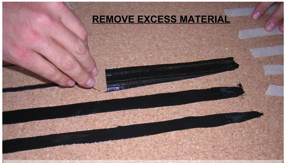
With a spatula or squeegee flatten and remove excess deck caulk material. Do not attempt to put this excess material into a groove, as it will trap air and you will have to return to repair the void which will show itself when sanding.
